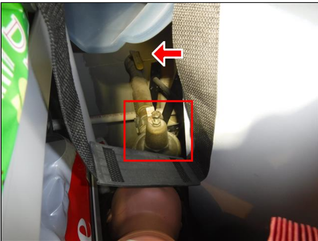
5.3 Item 3(Picture) 105 - Water pressure manifold and shutoff valve in the back utility closet.
