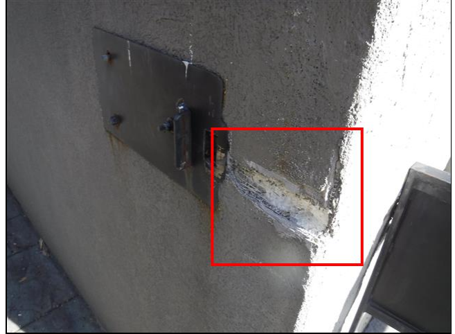
2.0 Item 2(Picture) 101- Exterior rear wall has been damaged by the gate lock.
