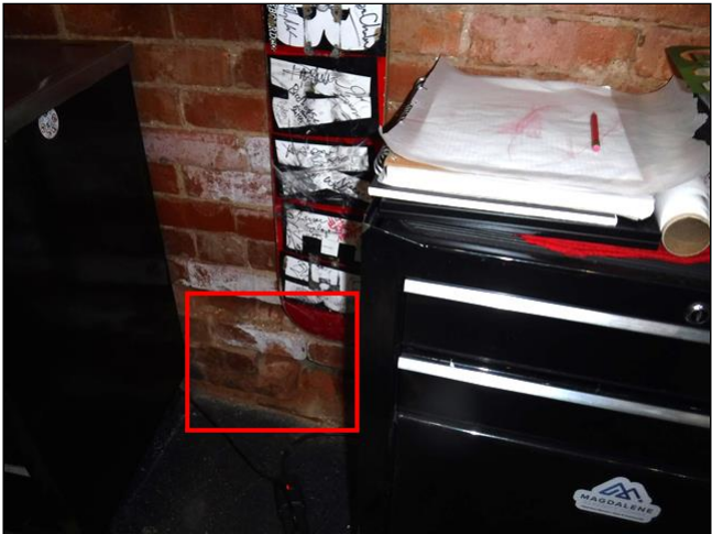
3.1 Item 2(Picture) 101 - Interior south brick wall shows advanced deterioration and efflorescence on the bottom half of bricks.
