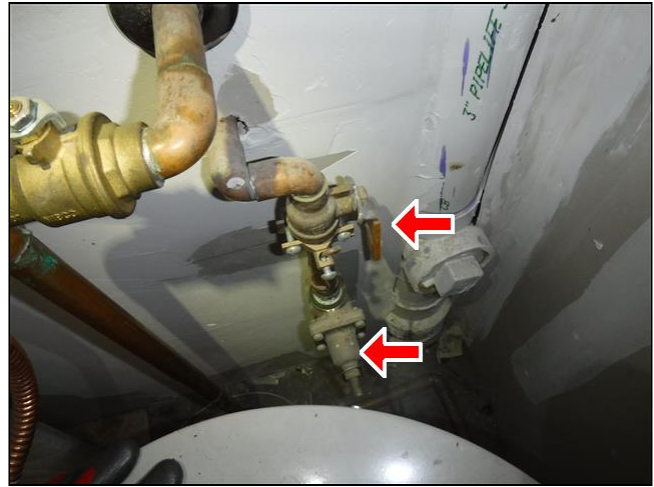
5.3 Item 2(Picture) 103 - Water pressure manifold and shutoff valve in the back utility closet.
