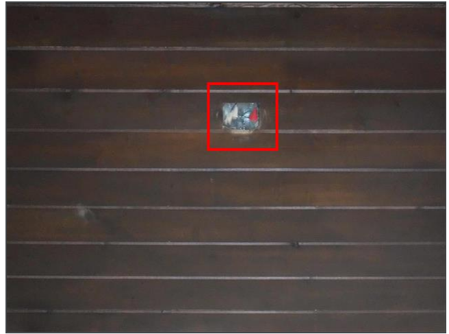
6.3 Item 2(Picture) 103 - Missing electrical box cover.
