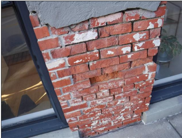
2.0 Item 3(Picture) Aged/Deteriorated bricks on the exterior of the building.
