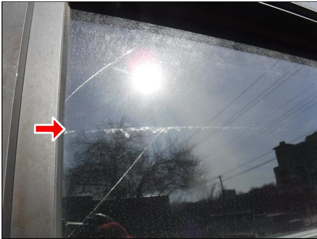
2.3 Item 1(Picture) 101 - Crack in the overhead patio door glass
