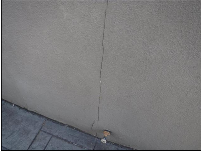
2.0 Item 1(Picture) 101 - Rear building EIFS is cracking at the seams.
