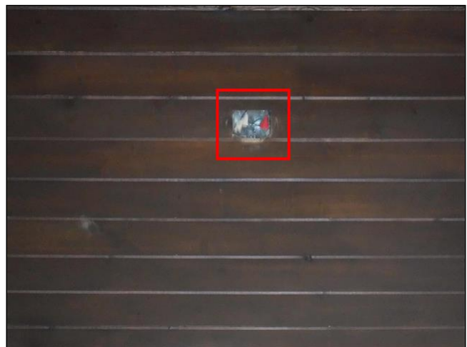
6.3 Item 2(Picture) 103 - Missing electrical box cover.
