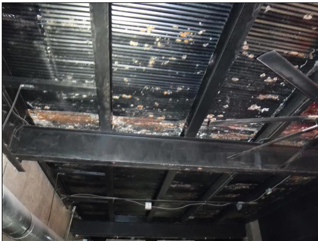
2.2 Item 1(Picture) 101 - Metal patio ceiling shows advanced deterioration and leaking.
