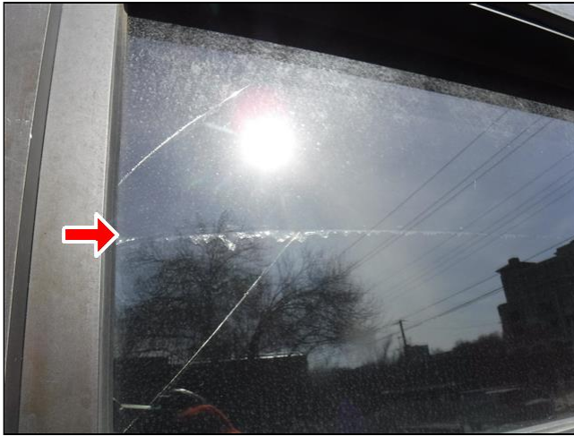
2.3 Item 1(Picture) 101 - Crack in the overhead patio door glass
