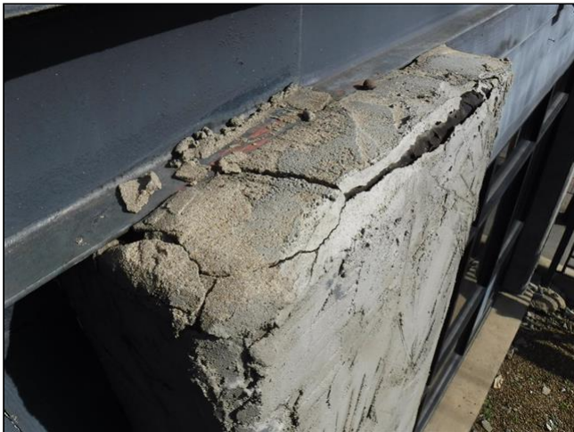
2.0 Item 5(Picture) 101 - Top concrete screeded pillars show advanced deterioration and is likely allowing water inside the column.
