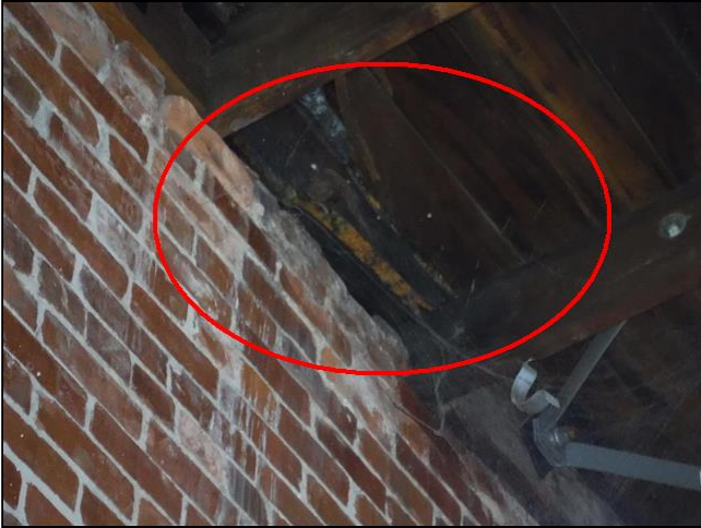
3.4 Item 1(Picture) Evidence of wood roof structure deterioration.
