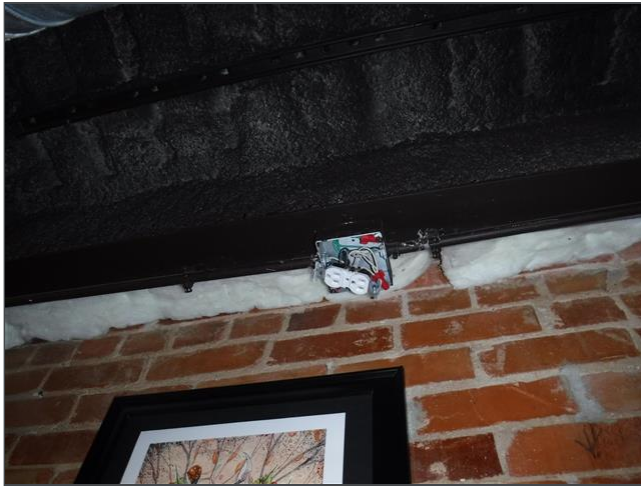
6.3 Item 1(Picture) 101 - Loose electrical receptacle
