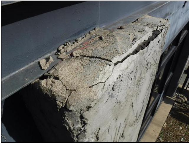
2.0 Item 5(Picture) 101 - Top concrete screeded pillars show advanced deterioration and is likely allowing water inside the column.
