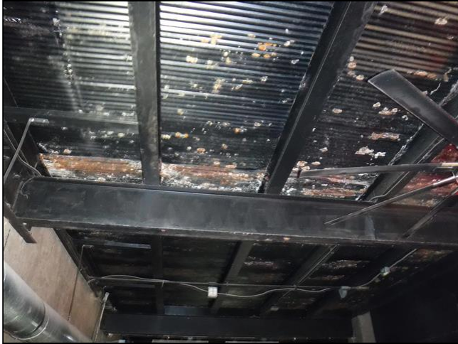
2.2 Item 1(Picture) 101 - Metal patio ceiling shows advanced deterioration and leaking.
