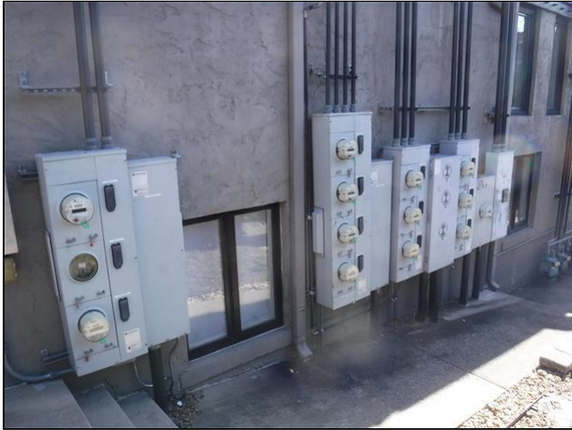
6.6 Item 1(Picture) Main Exterior Electrical Panels and Meters.
