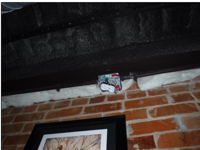
6.3 Item 1(Picture) 101 - Loose electrical receptacle
