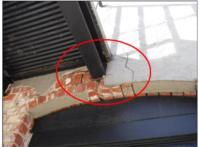
2.0 Item 4(Picture) Brick and concrete screed deterioration at the 2nd story patio on the front of the building.
