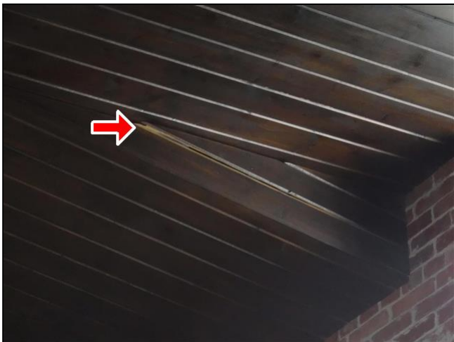
7.0 Item 1(Picture) 103 - Wood ceiling panel in the entry is loose.
