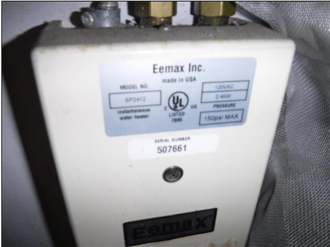
Shared hallway bathroom tankless water heaters x2 - unknown age.
