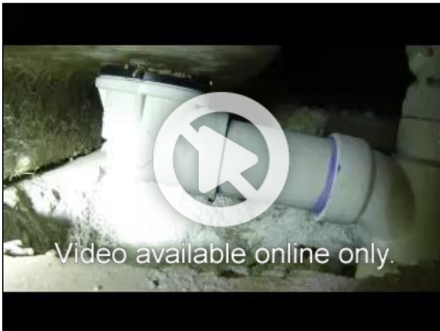
7.1 Item 1(Video) Water leaking out of the drain gasket for the master bath whirlpool tub.
