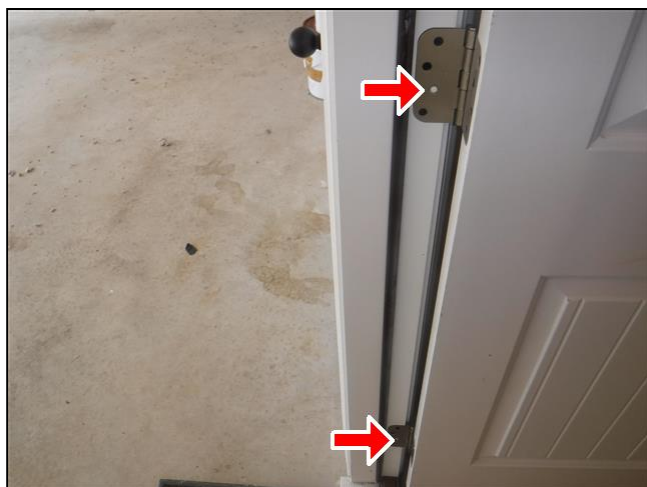
2.4 Item 1(Picture) Garage door hinges are missing mounting hardware.
