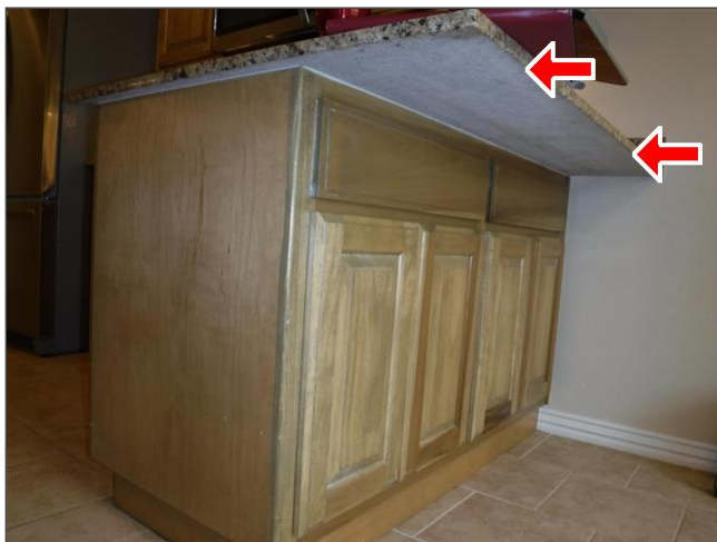
8.6 Item 1(Picture) Missing counter top supports.
