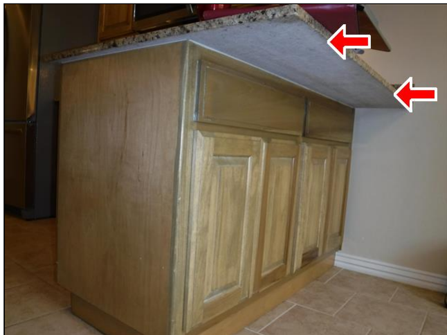
8.6 Item 1(Picture) Missing counter top supports.
