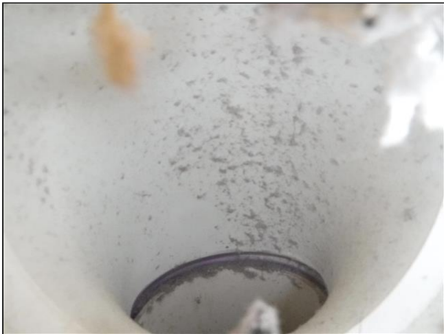
9.1 Item 1(Picture) No lint visible in the dryer vent.
