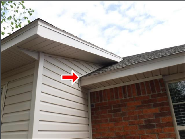
1.1 Item 2(Picture) Kick-out flashing recommended installation location. #1
