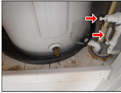
7.0 Item 2(Picture) Interior water shutoff and pressure manifold
