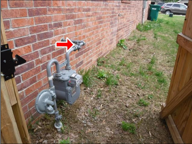
7.4 Item 1(Picture) Exterior gas meter and shutoff location.
