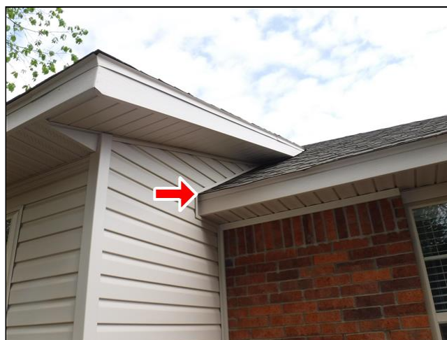
1.1 Item 2(Picture) Kick-out flashing recommended installation location. #1
