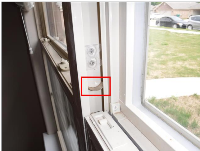
8.4 Item 1(Picture) NE bedroom window spring is disconnected
